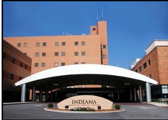
Figure 1 – Current Entrance to IRMC
